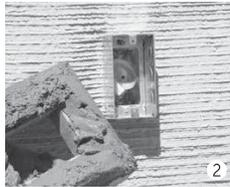
2 Apply mortar to back of electrical box stone or prepared substrate.
