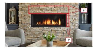
The area highlighted in red is a typical zone of risk related to excessive heat driven color change. Dimensions may vary slightly by manufacturer. Check with fireplace manufacturer to verify temperatures will not exceed 350° F.
